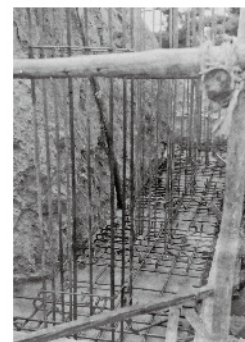
(c) 補強RC架構・基礎柱配筋
